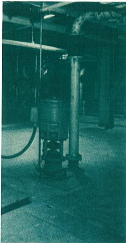
Shown above is one of four Nagle 6" Type YWS-R Frame 143-N pumps, each with an 11'4" setting. The water end was constructed of alloy HC-250 and the four pumps have been handling a total of 4,000 GPM of water and fly ash slurry since 1963 at a major power company.
