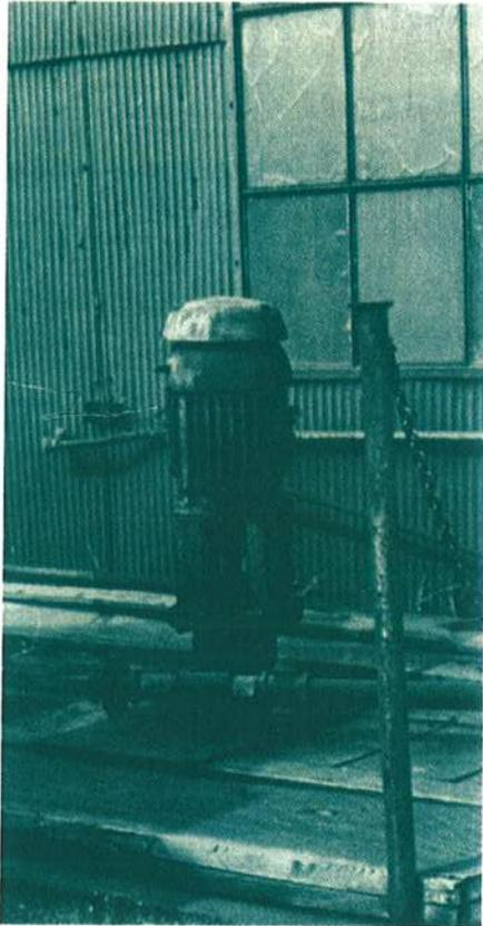
This Nagle 2 Type YWS-C Frame 71-HL pump with a 6'8" setting has been handling 100 GPM of carbide sludge from an acetylene generator in a Midwest metal working plant since 1962.
